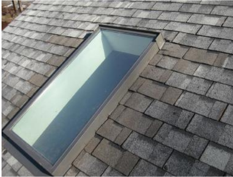
Recent repairs at skylight.
