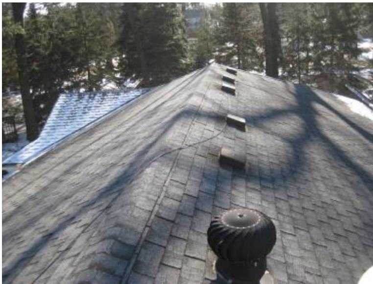
Overview of roof.
